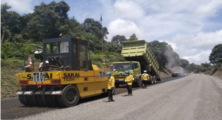
Hauling Road Upgrade
